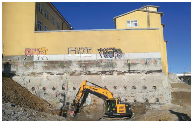
Figure 11. The underpinned building at final excavation level
