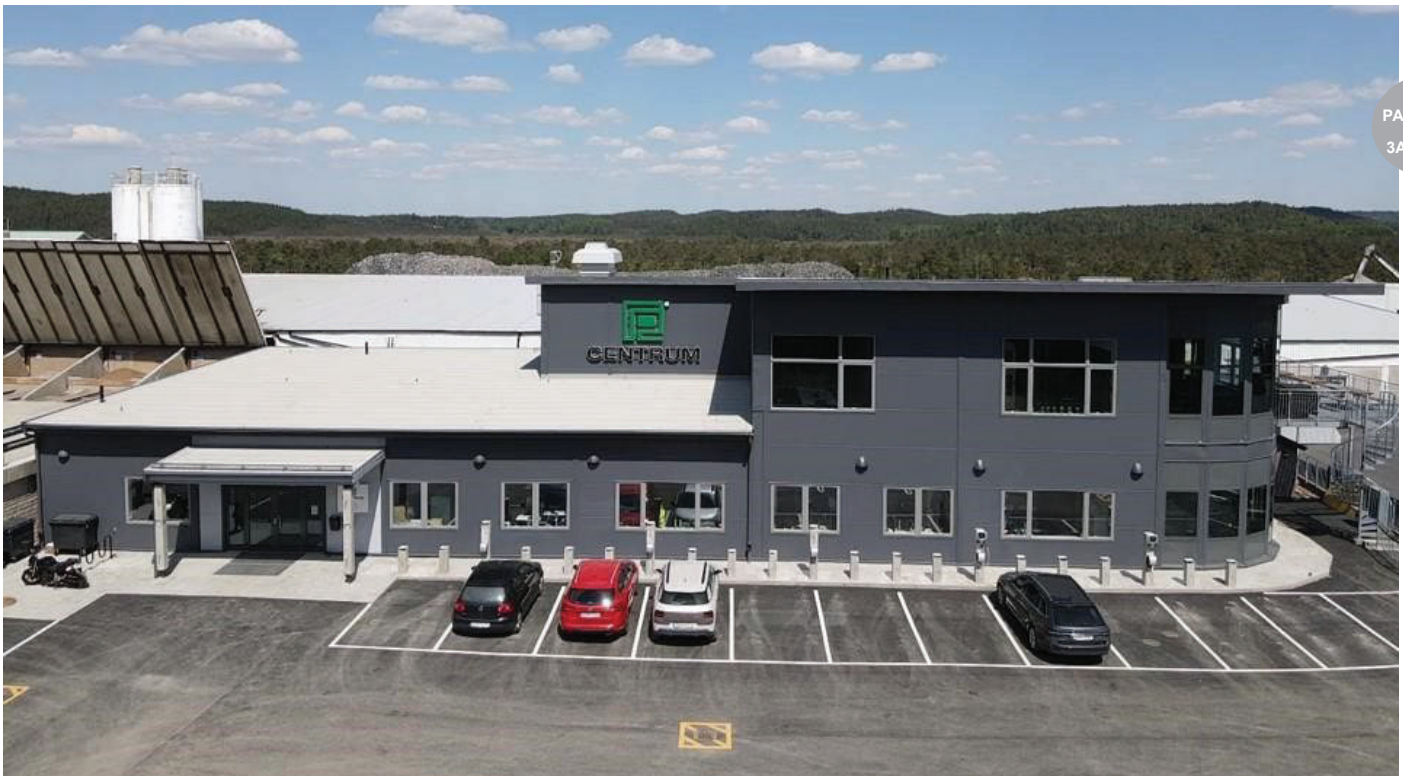
Figure 6 - Centrum Pile HQ, 2021, founded on 48 pcs. 15 meter precast energy piles. Property of Centrum Pile AB.
