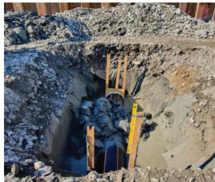
Figure 15. Partially excavated sample pipe
