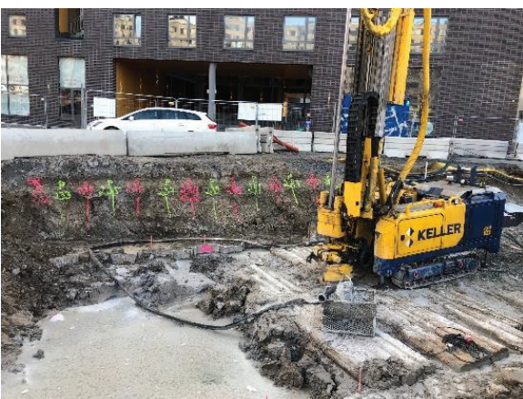
Figure 12 & 13. Impressions during execution of JG and excavation
