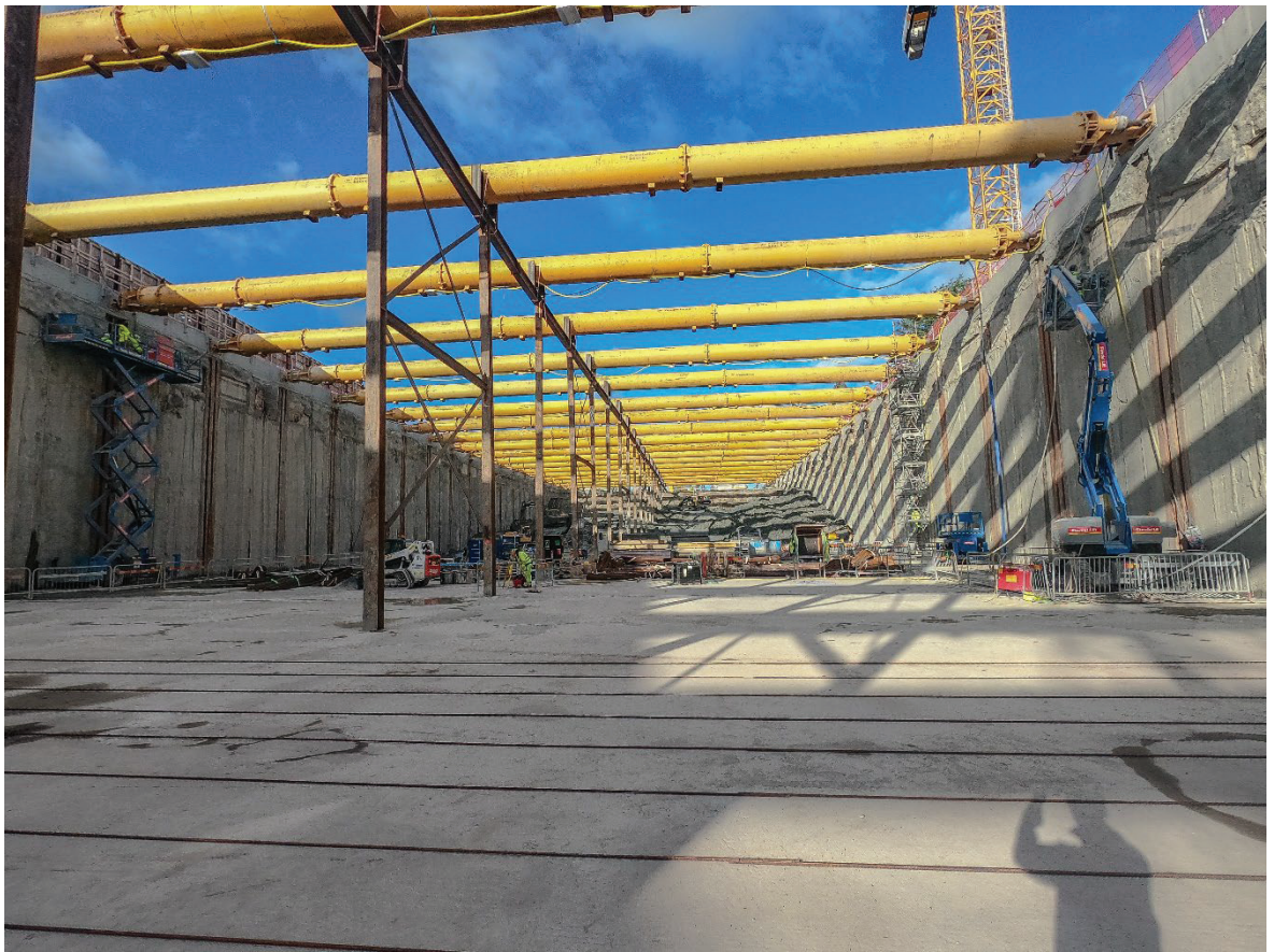
Figure 12. Construction pit after excavation
