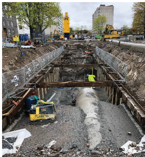
Figure 12 & 13. Impressions during execution of JG and excavation
