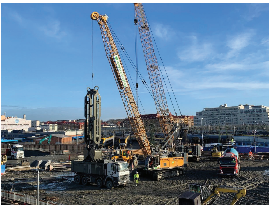
Figure 6. Machinery for excavation of diaphragm walls
